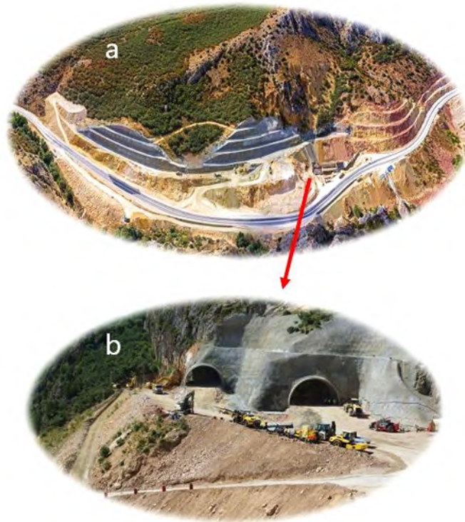
Figure 14. Tunnel entrances (a) starting from the steep slopes of Kırkdilim Canyon are constructed as right and left tubes (b). 33
