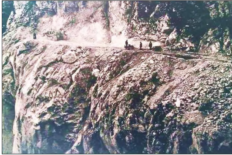
Figure 7. The first road construction work in Kırkdilim Canyon (1962) 25
